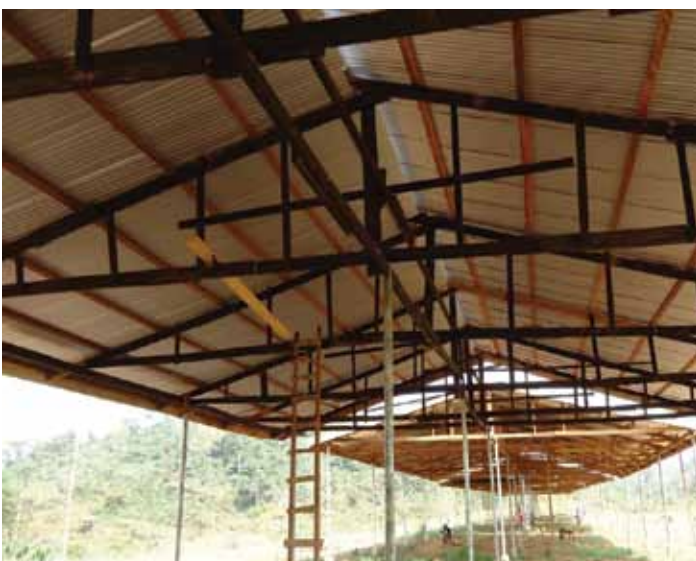
Construction of a new artisan market to relocate artisans
